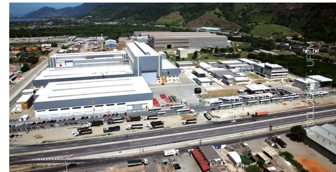
Steel Structure Manufacturing Unit (UFEM), Itaguaí - RJ
